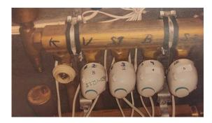
Möhlenhoff actuator with adapter ring for Kilimi's brass manifold (the valves are located under the manifold extensions).
